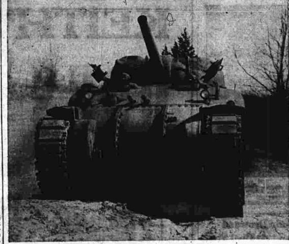
e with 75 mm. gun and a battery of machine guns. The M-4 has an all-cast body
